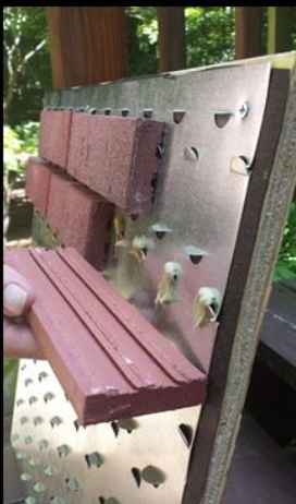
4.) Install Thin Brick
