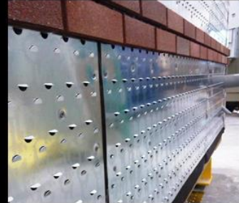
1.) Install BrickFast™ Panel
